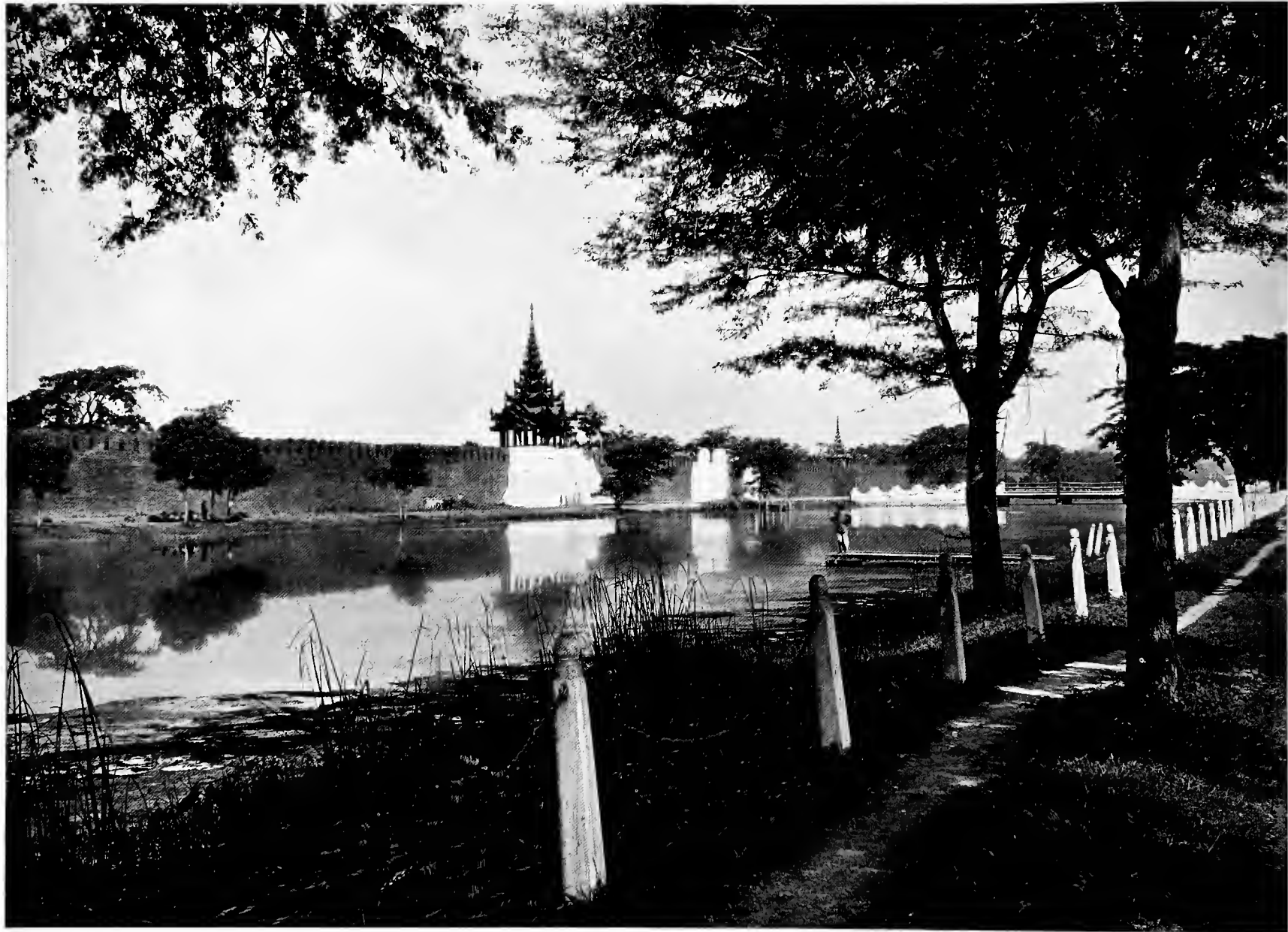
North Moat and Wall, Mandalay
